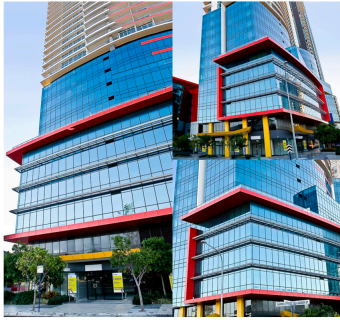
AGC Glass, AU 2017 Bears ultimate ocean front east spray. Invisible Shield was used to treat glass for long term protection against contaminants and permanent corrosion.
